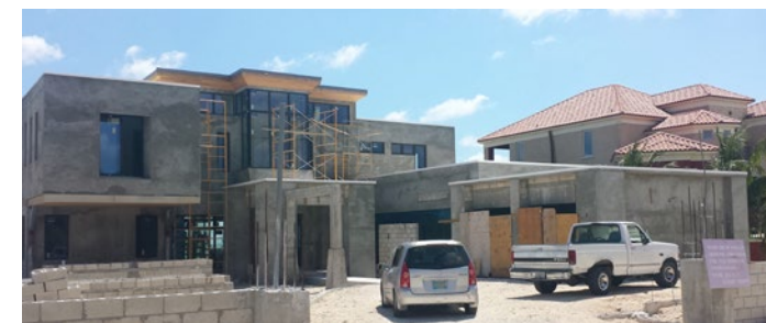
WHITE OCEAN ESTATE CONSTRUCTION
